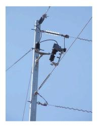
contact incidents. The switch to fiberglass materials assisted in insulation as well. Carbon Power and Light also implemented the suspension of conductors below the crossarm, which provides a perch area. These and other best practices are identified by the Avian Power Line Interactive Committee (APLIC) in its Avian Protection Plans Guidelines.
