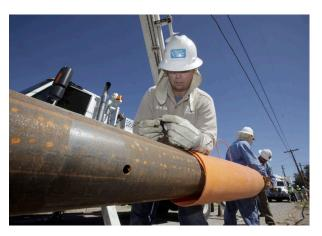
TEP uses greater mil thickness than the industry designed standards on the embedded portion of the pole, taking special care to understand the geotechnical aspects of the soils in order to avoid corrosion over the lifetime of the pole.
