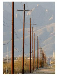
Since moving to steel poles almost exclusively, TEP has noted improvement of system reliability. Wind is the most severe natural power system problem on our system.
